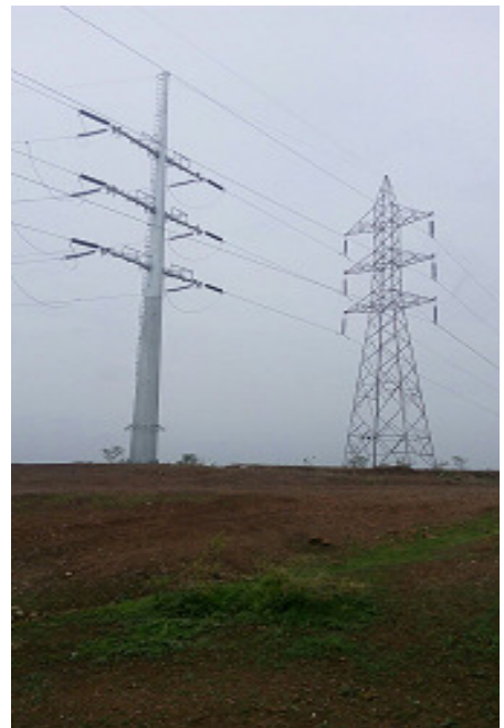
132 kV D/C, LILO Pole, MSETCL
