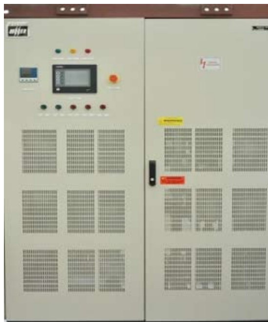
Fig. 4 : A view of In-house developed 500 kW PCS
